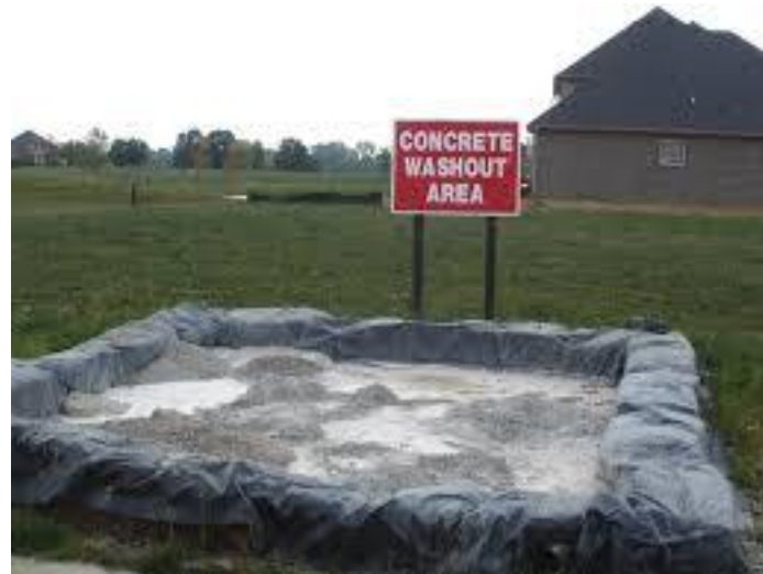
Figure 5.2 Example of temporary concrete washout area
